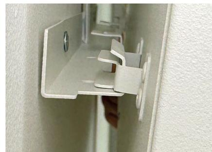
3. Attach the underside of the panel
